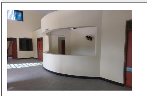
Figure 6: The Constructed EMD building at Morogoro RRH
