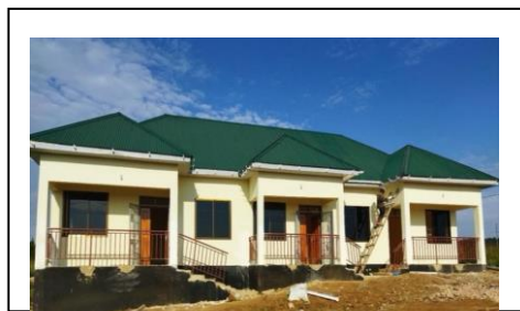
Figure 13 Staff house - Bukoba hospital
