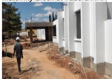
Figure 7: Construction of Maternity Block at Tabora RRH
