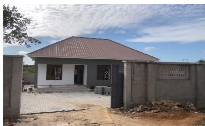
Figure 8: Construction of staff houses at Tumbi RRH
